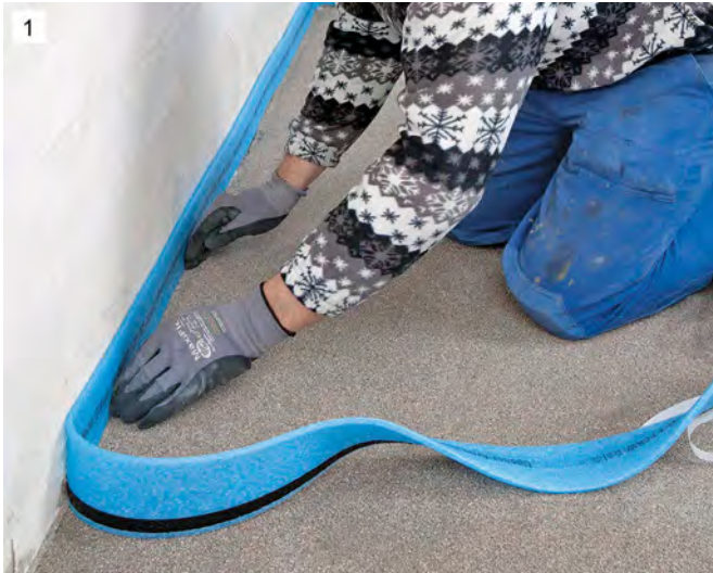
1) The Uponor Multi insulation tape with adhesive strips on the reverse are applied to all ascending structural elements such as walls, steps, etc. with no gaps.
