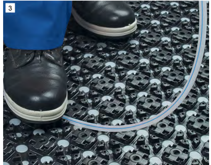
3) No tools are required for the installation of the Uponor Minitec Comfort Pipes. They are simply pressed into the studs of the foil elements at angles of 90° or 45°.
