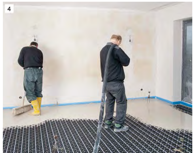
4) Finally, the levelling material only needs to be placed on the laid and finished Uponor Minitec surface and levelled with minimal coverage. The perforation of the foil elements ensures an optimal binding of the levelling material and substrate.
