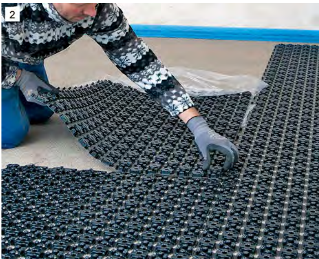
2) Then, the self-adhesive Uponor Minitec foil elements are laid out on the prepared substrate with gaps of approx. 5 cm between each one and are connected to each other with triangular studs.
