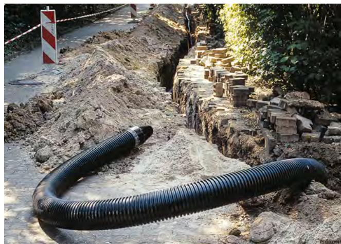
The flexibility of the Uponor Ecoflex pipes allows for problem-free adaptation on-site to almost any routing conditions. It is possible to route over or under existing lines, while obstacles can simply be avoided. Even laying the pipe system under a ground water table of 3 meter (0,3 bar) is permitted.
