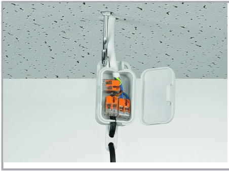
Pendant light connection in a suspended ceiling
