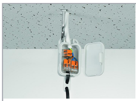
Pendant light connection in a suspended ceiling
