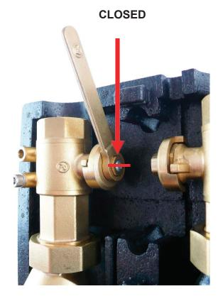
groove perpendicular to the flow direction
